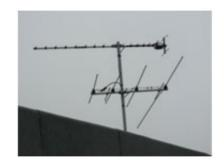
Antenna installed too close to roof
